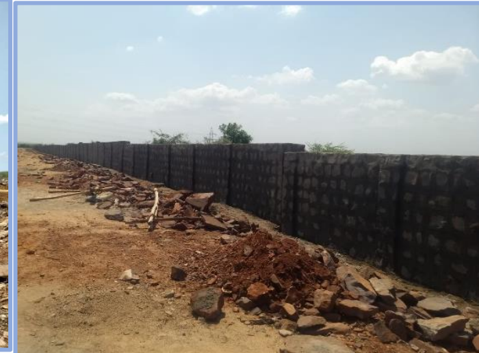
Compound Wall Construction
