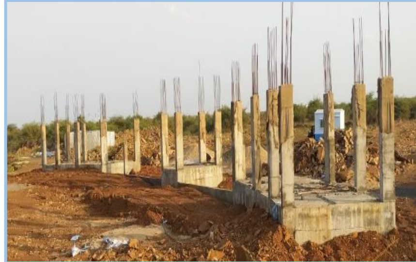
North Entrance Gate on Site
