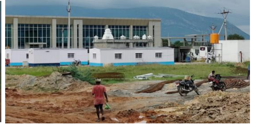
Civil Works commenced on October 2020
