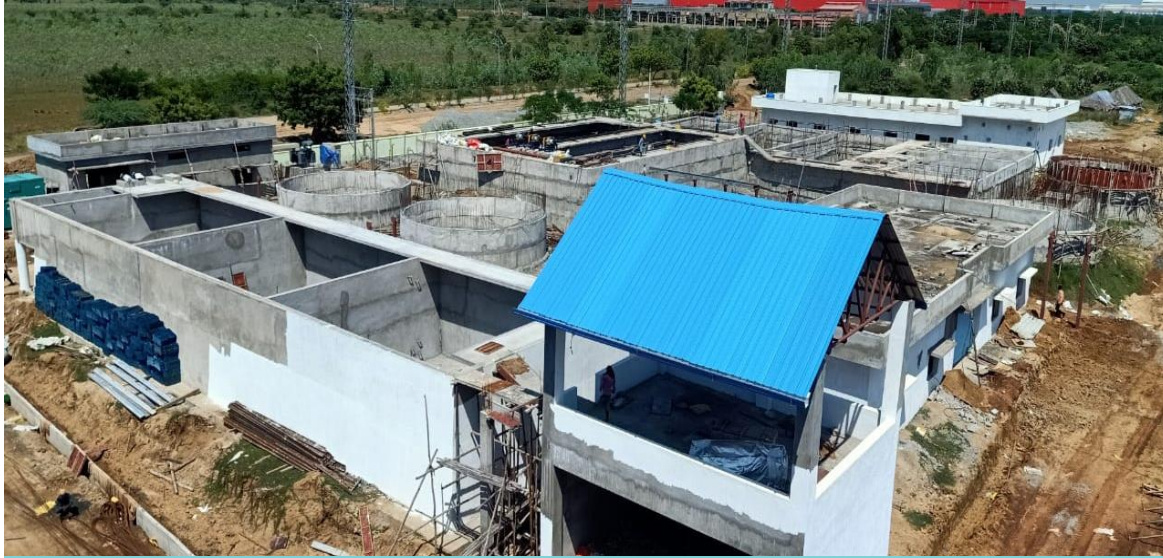
APIIC-01 : LTDS and centrifuge building and processing work
