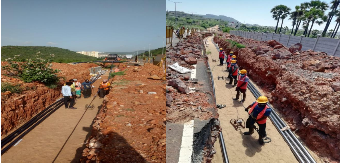
APTransCo./01 : Laying of Underground Cable at Kapuluppada
