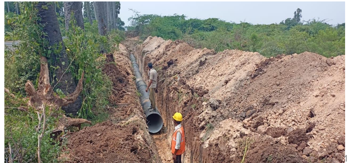
APIIC-05 : Laying of 700mm DIA DI K-9 Pipe along Rapur-Gudur-Krishnapatnam
