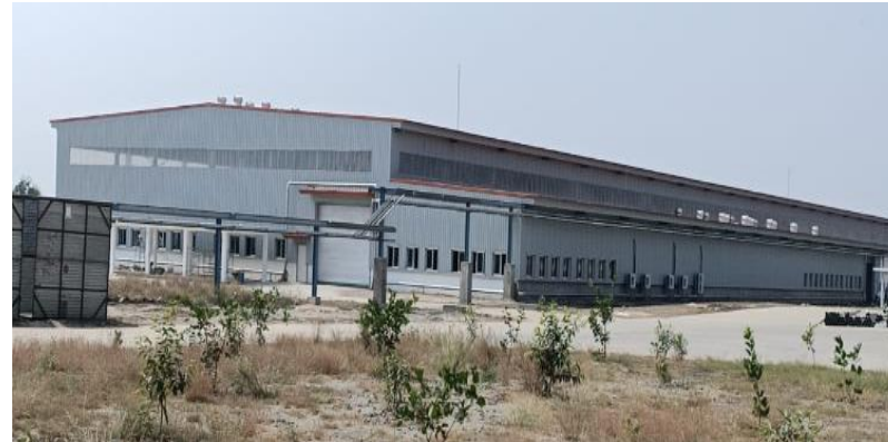
Civil Works completed for Machine Shop on March 2020
