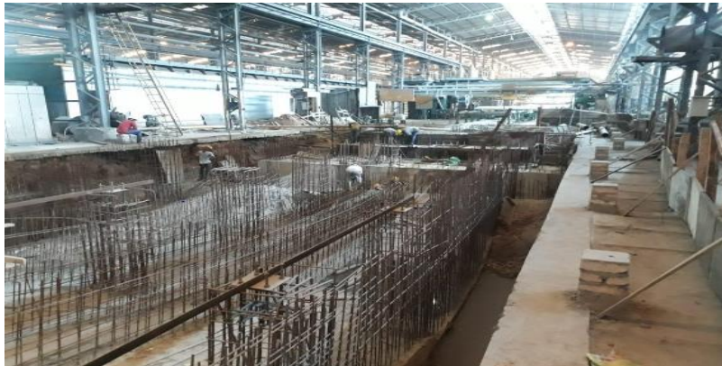
Civil Works commenced on March 2020
