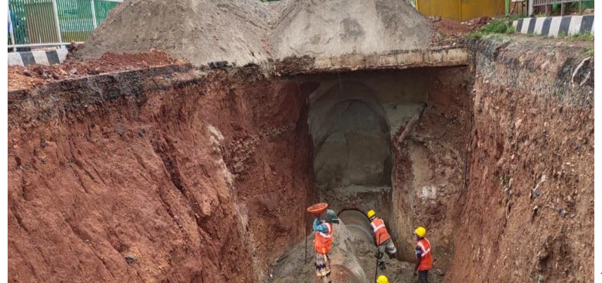
GVMC/02 : Gravity Main Lowering work : 24*7 Water Supply Project
