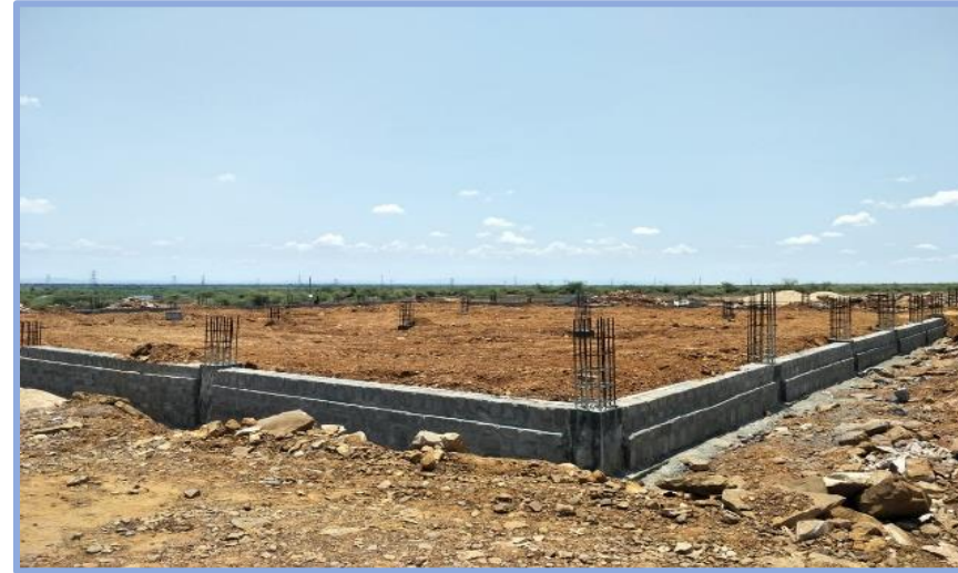
Project Office Foundation at project Site
